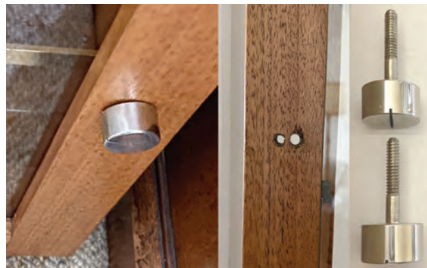
Lower bolt Holes Bolts Figure 9-1 The door
